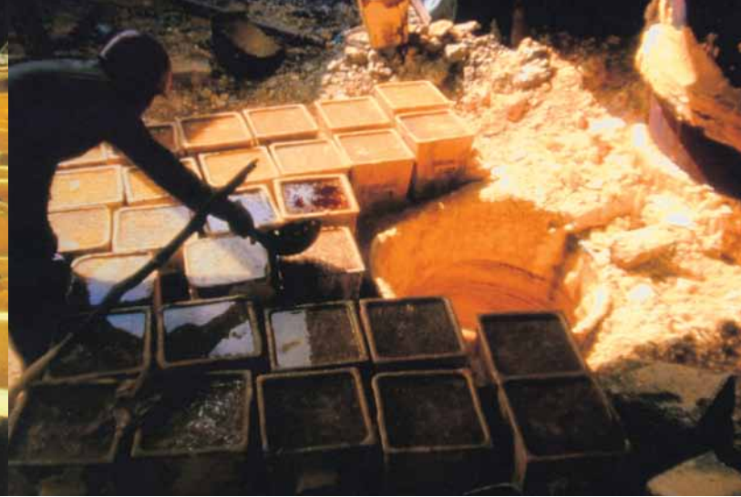
早期陽明山國家公園的大油坑採硫過程。左圖為製硫廠 / 陽管處提供 The process of sulfur mining at Dayoukeng in YMSNP back in the era of mining industry. The picture on the left shows a sulfur factory./ Provided by YMSNP Headquarters
